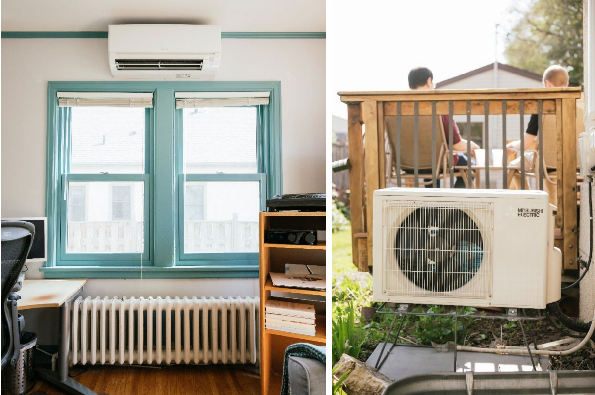
Figure 2. Example of a ductless ASHP
