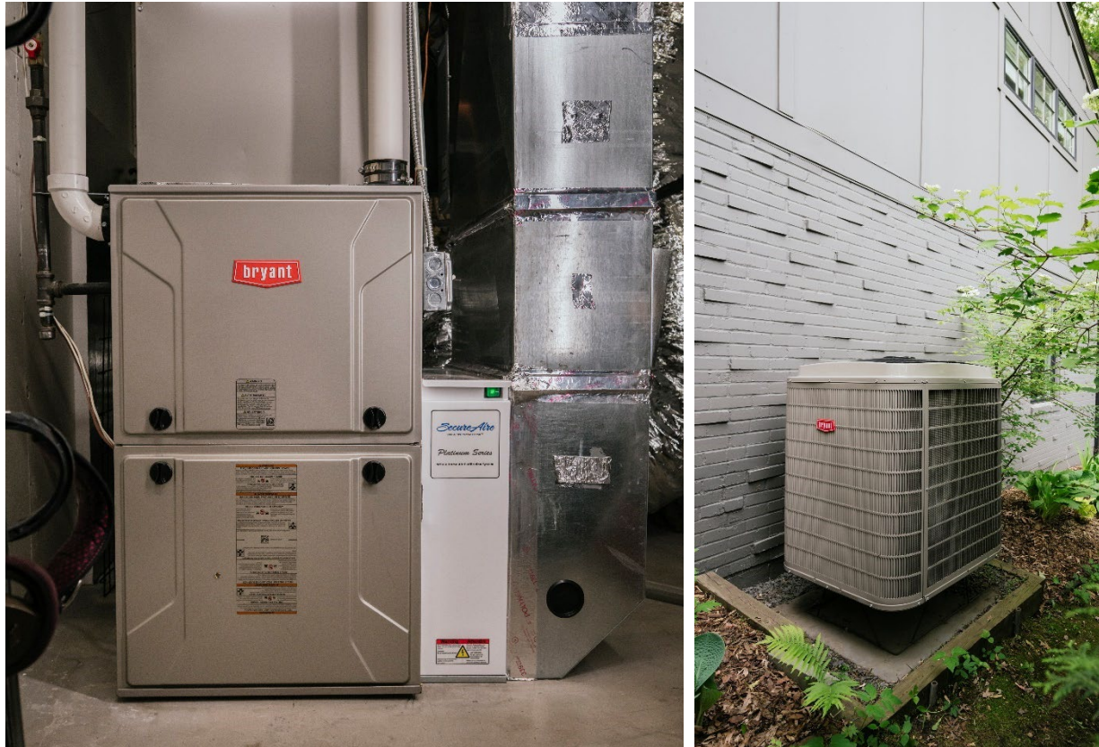
Figure 3. Example of a ducted ASHP
