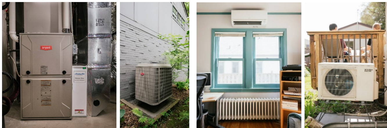
Figure 1. Exterior and interior equipment of ducted (left) and ductless ASHP (right)
