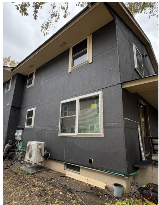
Figure 6. HPW demonstration site with co-installed continuous exterior insulation (CEI), Minneapolis, MN
