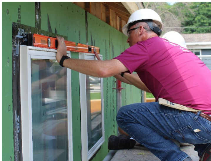
Figure 7. HPW demonstration site with Twin Cities Habitat and Andersen Windows, Maplewood, MN
